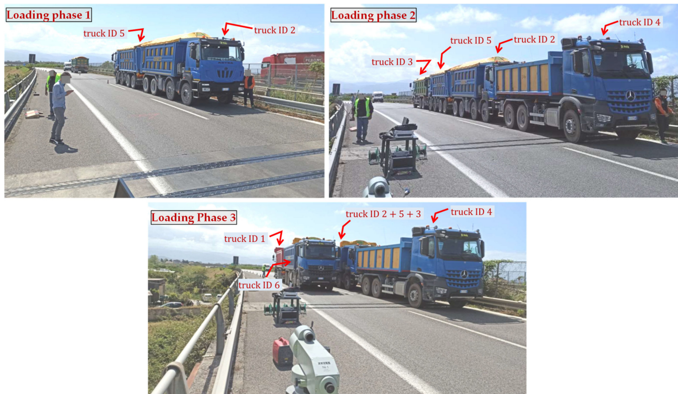
Figure 14. Photographs of static load tests in three subsequent phases for the roadway from Palermo to Messina.
