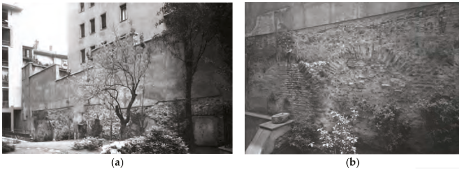
Figure 2. Photographs of the remains of the external wall of the circus visible in a private garden of a building in via Vigna 1: (a) the entire portion of the remains; (b) a detail of the arches sustaining the podium visible on the wall (courtesy of Ministero dei beni e delle attività culturali e del turismo).
