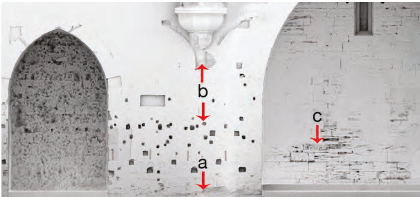
Figure 4. 2D raster from an environmental occlusion generated in 3D: (a) loss of material; (b) holes and alterations of the stone; and (c) disintegration of stone.
