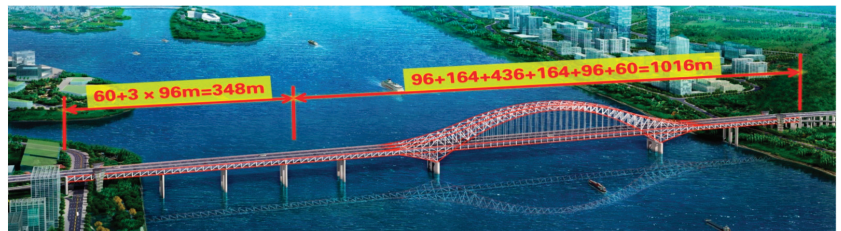
Figure 2. General layout of Guangzhou Mingzhu Bay Bridge.
