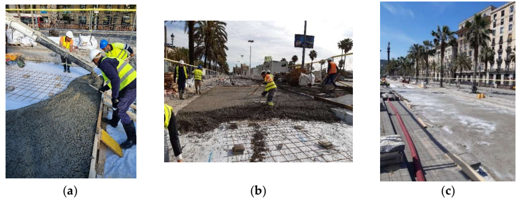
Figure 6. On-site concrete laying (a), compaction (b) and curing process (c) of the concrete.
