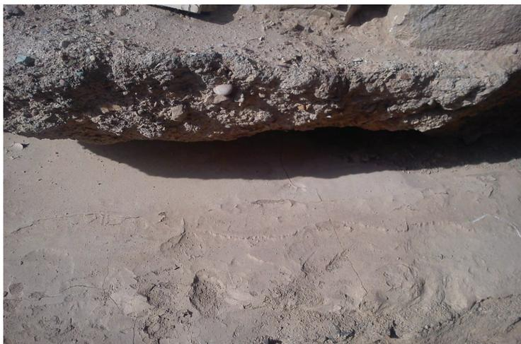
**Figure 22.** Bridge scour in bridge No. 5.
