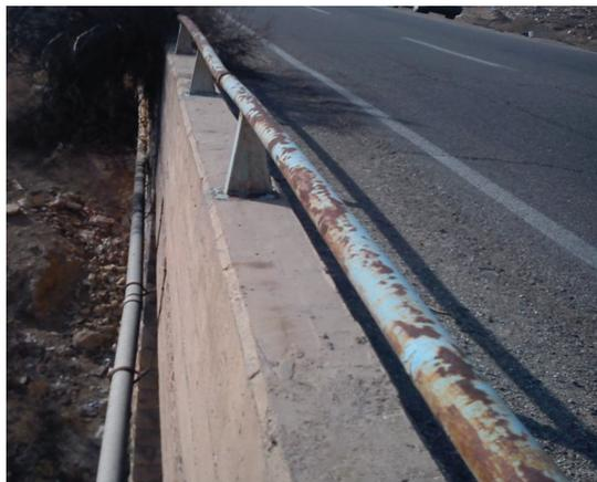
Figure 18. Safety and drainage issues in bridge No. 4.
