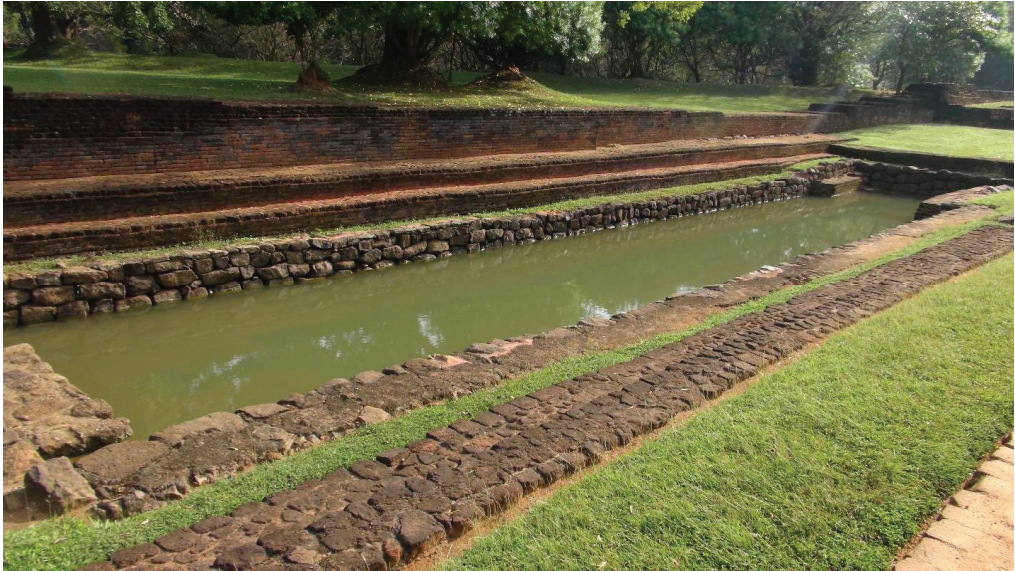
Figure 3. A water storage tank in the Sigiriya complex, Photo courtesy: Kenichi Matsui.
