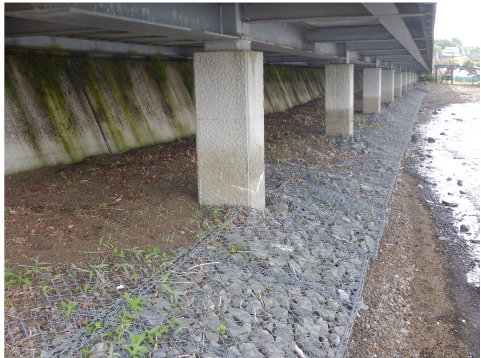
Figure 7. Reclamation of the lake's shoreline and parking lot construction. Photo taken on 19 June 2022, when the lake water level was 2.26 m.
