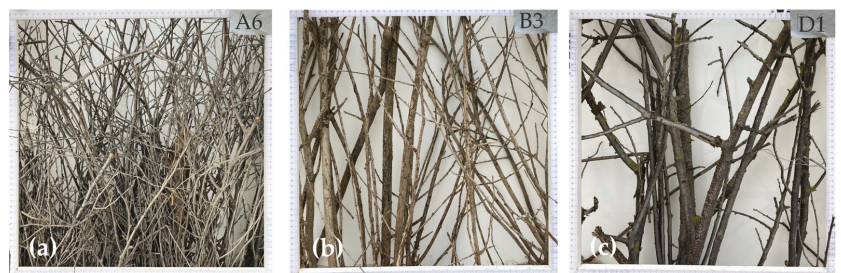
Figure 6. (a) Standardized section of the sand trapping fence with 5 bb/m, (b) standardized section of the sand trapping fence with 3–4 bb/m, (c) standardized section of the sand trapping fence with 2 bb/m.
