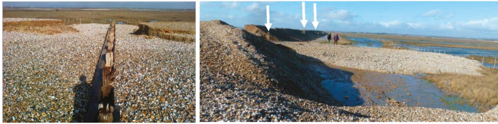
Figure 11. (Left) Photo along groyne between profiles 53 and 54 taken on 18 February 2014 showing overwashing guided by the groyne; (Right) Photo looking west along the access path behind the barrier with overflow fan along profile 42 behind the groyne. Arrows point to the landward termination of the groyne. Photo taken following the February 2014 storms.
