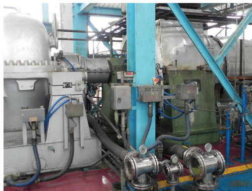
Figure 8. The data acquisition platform.
