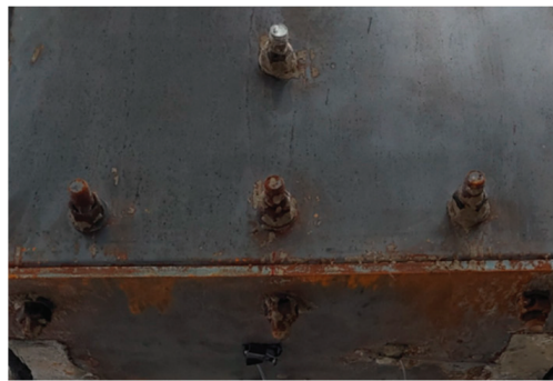
Figure 12. The side plate and bottom plate after a flexural test.
