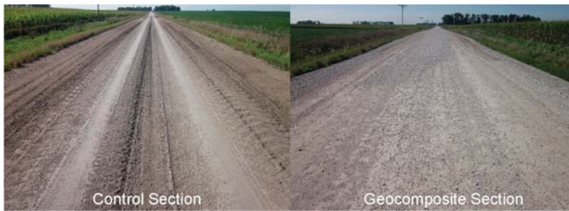
Figure 9. Surface conditions of the unpaved road sections after a heavy rainfall (photos taken on 2 September 2015).
