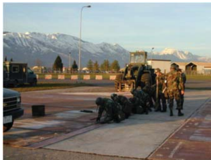
Figure 1. Anchoring the fiberglass mat.
