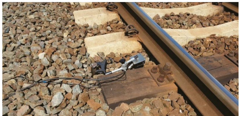
Figure 7. Measuring station—jumping change in the stiffness of the surface—access to the railway viaduct at km 88,882 LK No. 272.
