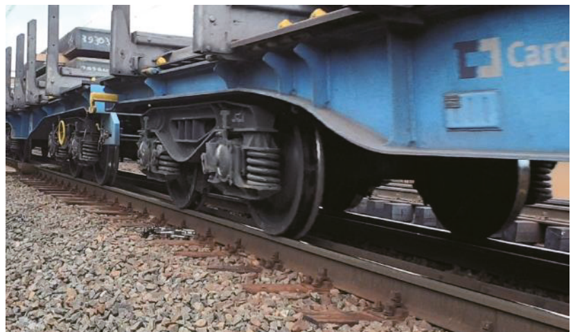
Figure 9. Railway viaduct at km 88,882 LK No. 272—measurement of the vertical displacement of a rail dynamically loaded with a freight train.
