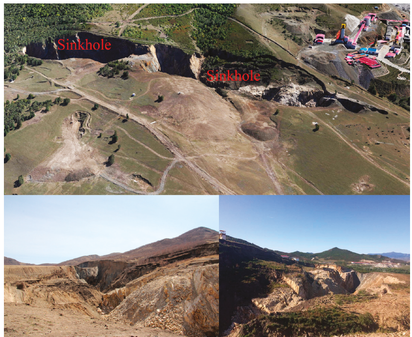
Figure 6. The aerial view of surface collapse.
