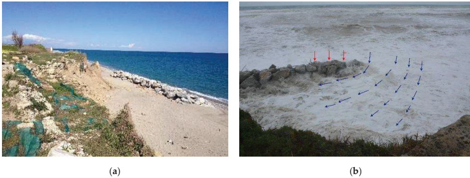
Figure 7. (a) Barrier made in January 2014. (b) Storm of February 2014 (blue arrows) that crosses the barrier (red arrows).
