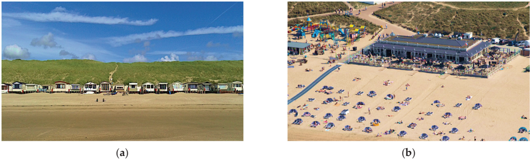
Figure 1. Buildings at beach–dune interface on the (a) Egmond beach, and (b) Zandvoort beach ( https://www.hollandluchtfoto.nl (accessed on 1 December 2021)), The Netherlands.
