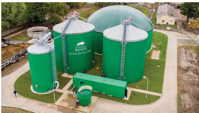
Figure 2. 500 kW biogas plant at Przybroda PULS experimental farm.
