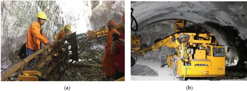
**Figure 25.** Mechanized installation of the arches. (a) Assembled arches near the ground and (b) the installation of upper bench arches.
