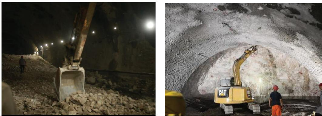
**Figure 24.** The preparation before construction. (a) Road surface treatment and (b) the overbreak and underbreak treatment.
