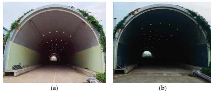
**Figure 2.** Tunnel appearance and decoration. (a) Sidewalls with energy-storage and luminescent coating, (b) sidewalls with gray cloth.
