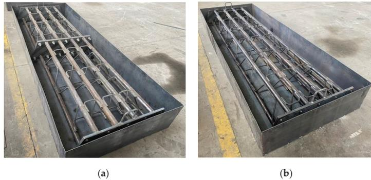
**Figure 3.** Before pouring of the spatial reticulated grid components. (a) The bolted end-plate joint component and (b) the jointless component.
