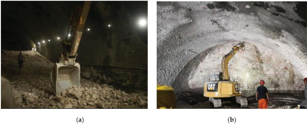
**Figure 24.** The preparation before construction. (a) Road surface treatment and (b) the overbreak and underbreak treatment.
