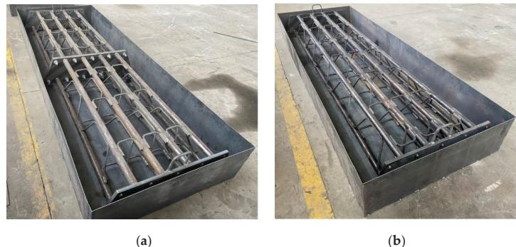
**Figure 3.** Before pouring of the spatial reticulated grid components. (a) The bolted end-plate joint component and (b) the jointless component.
