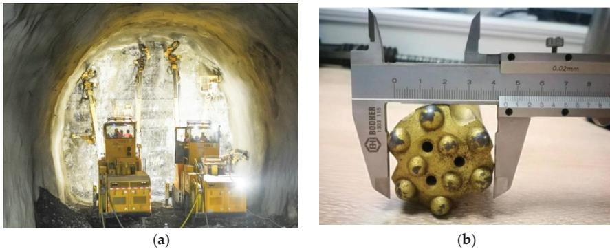
**Figure 4.** Field collection of the drilling parameters. (a) Blasting hole drilling in the tunnel face; (b) the cemented carbide bit.
