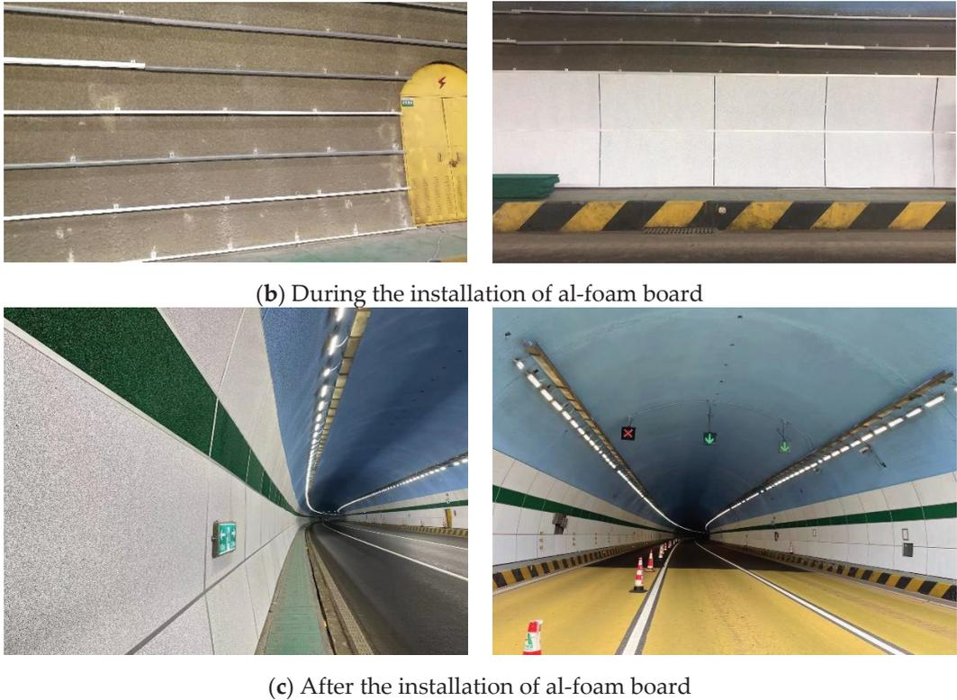
**Figure 12.** Comparison of the effect before and after installation of the al-foam board.
