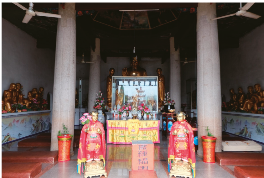
Figure 11. The petal-shaped corrugated stone pillars of four segments used in the main hall of Baoen Temple. Photograph by authors.
