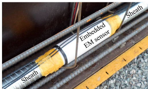
Figure 3. Installation of an embedded EM sensor.
