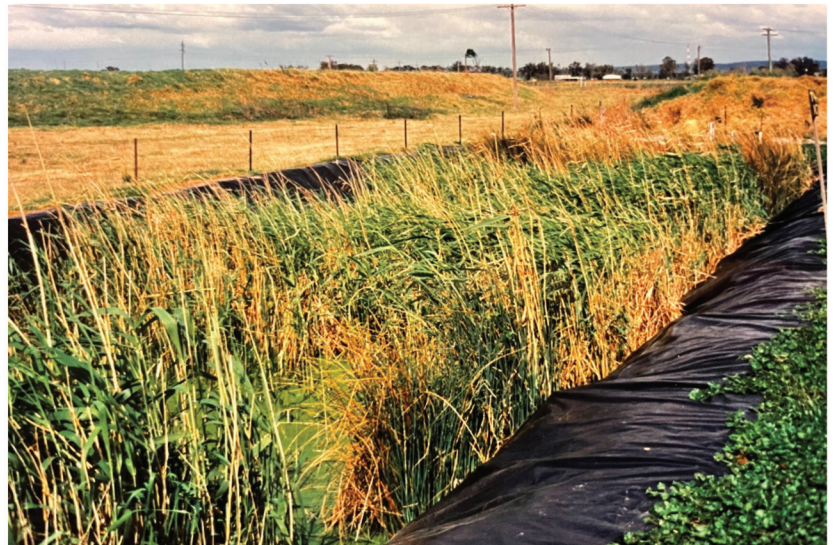
Figure 17. Experimental HF CW at the University of Western Australia, Hawkesbury. Photo Jan Vymazal.
