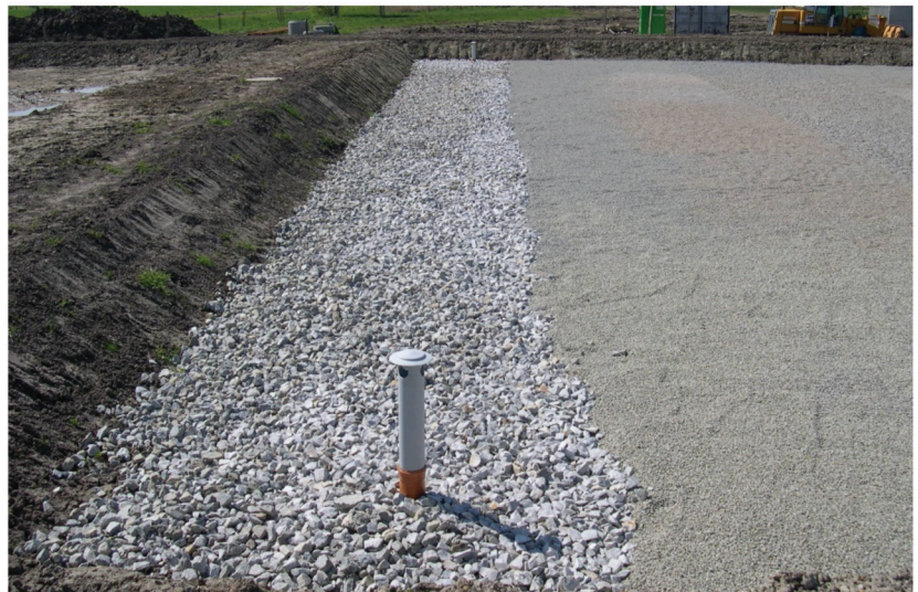
Figure 8. Distribution zone filled with large stones and the filtration bed filled with crushed rocks (4–8 mm) before planting. HF CW Čejkovice, Czech Republic. Photo Jan Vymazal.
