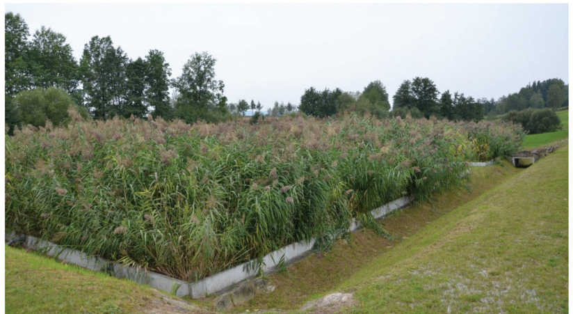
Figure 12. Down flow vertical constructed wetlands planted with Phragmites australis . Oberwindhag, Austria. Photo: Jan Vymazal.
