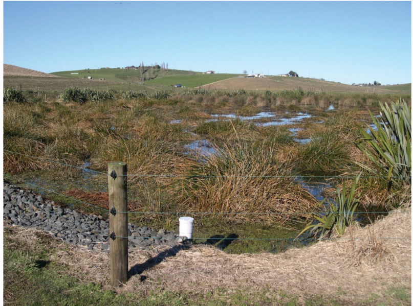
Figure 5. Surface flow CW with emergent plants ( Eleocharis sphacelata , tall spikerush). Otorohanga, New Zealand. Photo Jan Vymazal.
