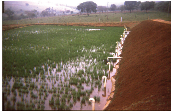
Figure 13. Vertical up flow constructed wetlands planted with rice ( Oryza sativa ) called “filtering soil”, in Piracicaba, Brazil. Photo Jan Vymazal.
