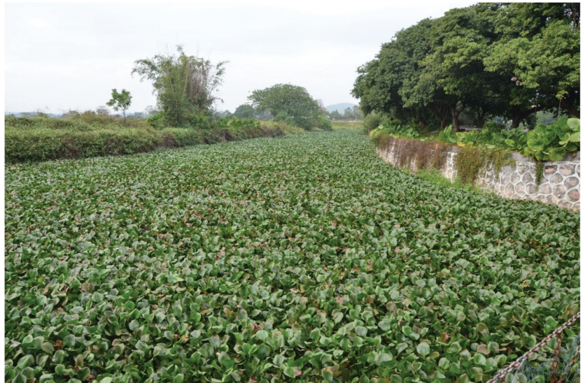
Figure 1. Surface flow constructed wetlands with Eichhornia crassipes (water hyacinth) in Langtou near Guangzhou, China. Photo Jan Vymazal.
