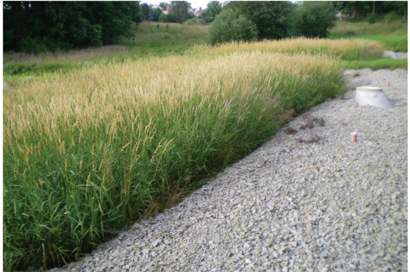
Figure 9. Constructed wetland with a horizontal subsurface flow. Roseč, Czech Republic. Photo Jan Vymazal.
