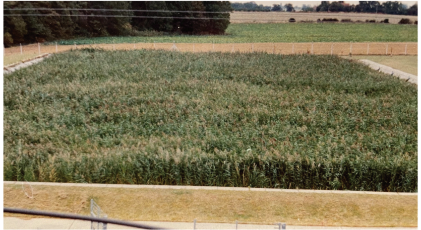
Figure 15. Horizontal subsurface flow CW, Freethorpe, United Kingdom, for 900 PE. The early CWs were built as a single bed. Photo Jan Vymazal.
