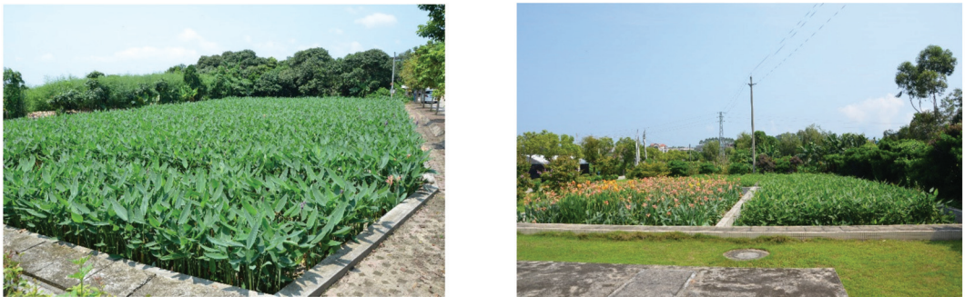
Figure 18. Constructed wetlands with horizontal subsurface flow, planted with Thalia dealbata (left) and Canna indica and Thalia dealbata (right) in Quangdong Province near Guangzhou. Photo Jan Vymazal.
