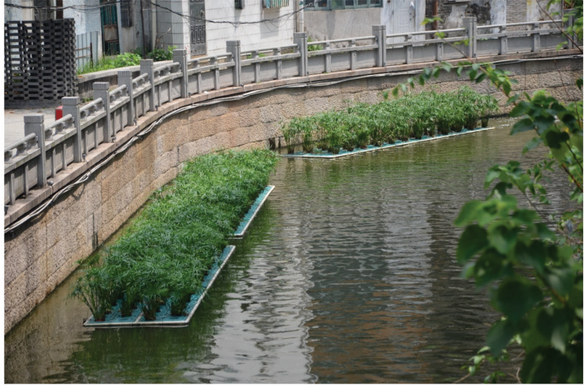
Figure 6. Floating constructed wetland planted with Cyperus alternifolius . Ningbo, China. Photo Jan Vymazal.
