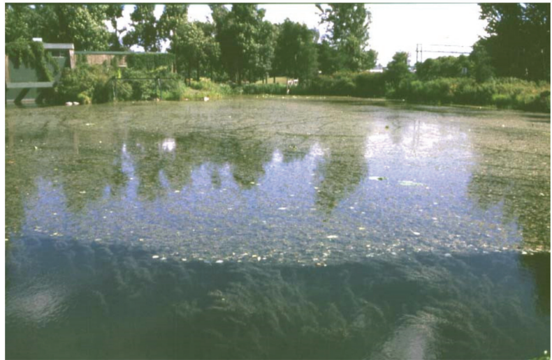
Figure 4. Surface flow CW with submerged macrophytes (mostly Myriophyllum spicatum , watermilfoil) in Montréal, Canada. Photo Jan Vymazal.
