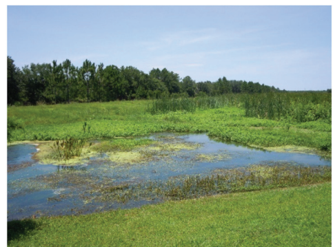
Figure 16. Surface flow CW at Ironbridge. Tertiary treatment for the city of Orlando, Florida. Photo Jan Vymazal.
