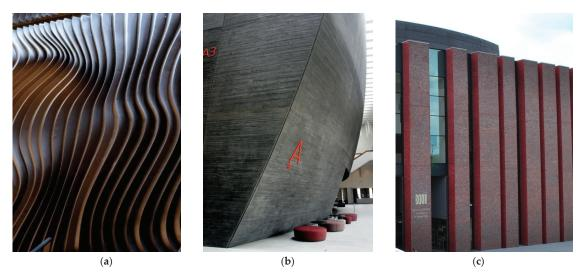
Figure 5. Polish National Radio Symphony Orchestra House, Katowice, 2014, arch. Konior Studio. (a) The inner precast concrete cladding of the main concert hall. Source: M. Charciarek [33]; (b): The inner cast concrete layered wall of the main lobby, (photo by M. Celadyn); (c): Main entrance. Source: https://commons.wikimedia.org/wiki/File:Katowice\_05.15\_NOSPR\_2.JPG (accessed on 31 May 2021), photo by M. Mróz.
