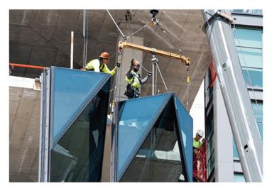
**Figure 5.** Several workers working at height during the CWM installation process (facade installation in Solar Carve Tower, New York. Facade engineered and manufactured by Focchi Group; photo by Timothy Schenck).
