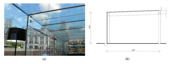
**Figure 20.** The Costa Coffee London: (**a**) view inside the glass pavilion (photo by the author); (**b**) glass frame geometry (figure by the author).
