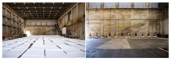
**Figure 15.** The 10 fabric strips were first unrolled on the ground and connected to the cables (**a**). The entire system was later lifted into the final position through a set of hand-operable winches located at the ground level (**b**). Photos by Shuaizhong Wang.
