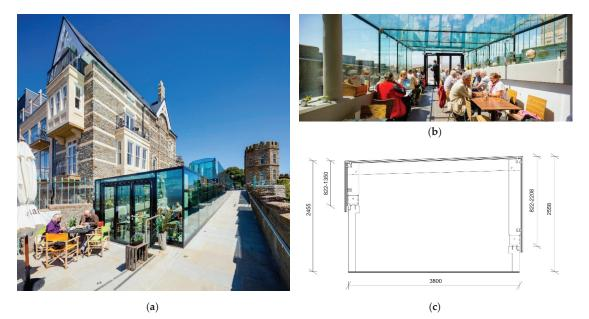
**Figure 21.** The Clevedon Pier Visitor Center: (**a**) view of the tearoom pavilion (© Fotohaus); (**b**) view inside the pavilion (© Fotohaus); and (**c**) glass frame geometry (figure by the author).
