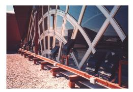
**Figure 24.** Semicircular opening and projecting overhang at the extreme of the central conoid of the School of Engineering of Seville.
