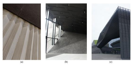
Figure 3. International Congress Centre, Katowice 2015, JEMS Architects. (a) The sound absorbing wall cladding in the multifunctional space, (photo by A.K. Kłosak); (b) fragment of the main hallway, (photo by M. Celadyn); (c) main entrance, (photo by M. Celadyn).
