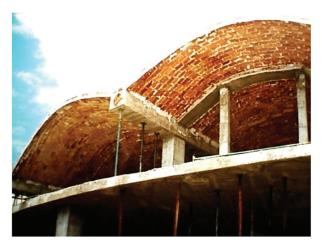
Figure 27. Vault pieces are constructed in hollow thin brick with steel mesh for reinforcement and attached to a concrete frame.
