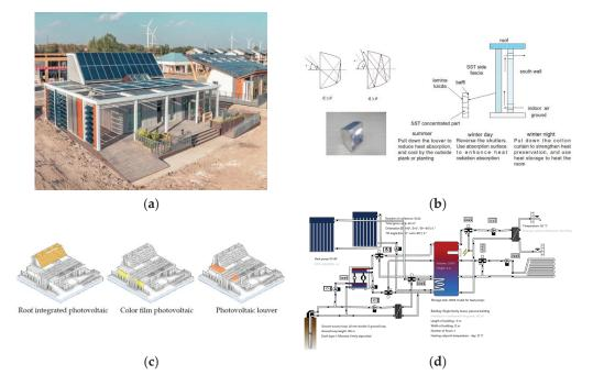
Figure 10. Main results of the T&A House. (a) Assembled T&A House. (b) SST wall. (c) PV used. (d) Ground source heat pump system.
