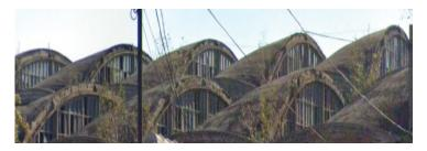
Figure 21. Close-up of the array of the conoids still standing after 64 years without maintenance.
