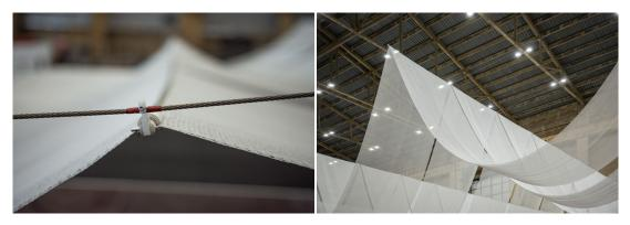
**Figure 13.** (a) The detail of the joints' final expression; (b) The joints become invisible from a distance. Photos by Shuaizhong Wang.
