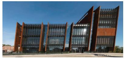
**Figure 3.** The south and west façade of the ECS, with structural walls which deviate from the vertical by 6.5°. The façades of the ECS are covered with 5 mm thick corten plates (photo by Wojciech Kryński).
