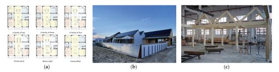
Figure 9. Main results of the Pixel House. (a) Changeable modules. (b) BIPV and PV fence. (c) Prefabricated wooden structure.
