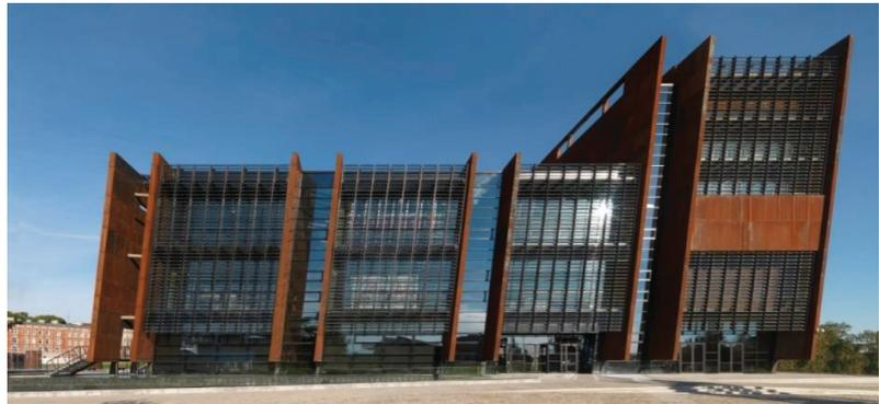
**Figure 3.** The south and west façade of the ECS, with structural walls which deviate from the vertical by  $6.5^\circ$ . The façades of the ECS are covered with 5 mm thick corten plates (photo by Wojciech Kryński).
