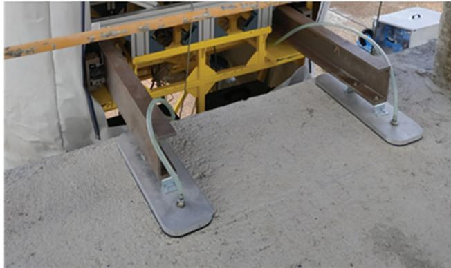
**Figure 8.** Stabilizer attaching the robot platform to the concrete slab (photo: José David Jiménez-Vicaria).
