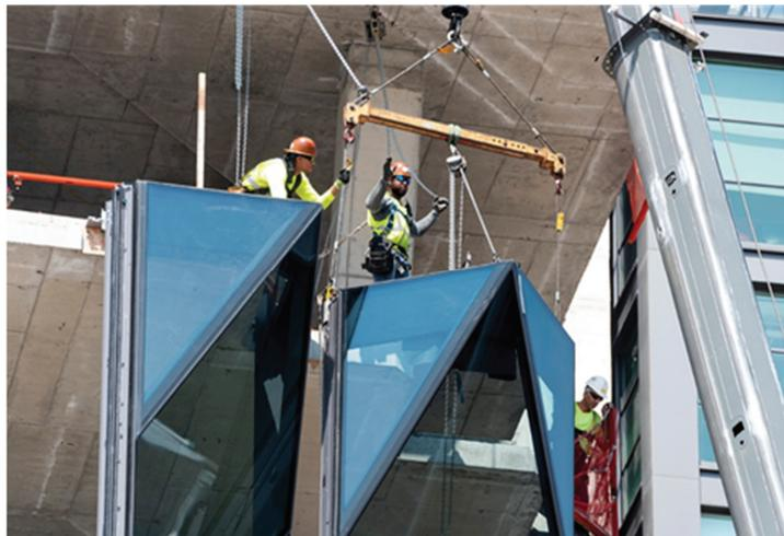
**Figure 5.** Several workers working at height during the CWM installation process (facade installation in Solar Carve Tower, New York. Facade engineered and manufactured by Focchi Group; photo by Timothy Schenck).
