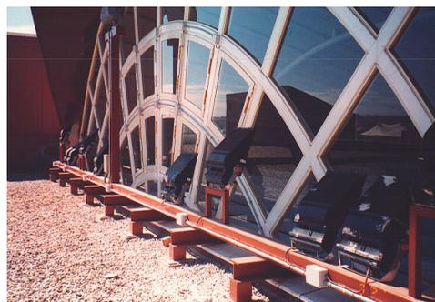
**Figure 24.** Semicircular opening and projecting overhang at the extreme of the central conoid of the School of Engineering of Sevilla.
