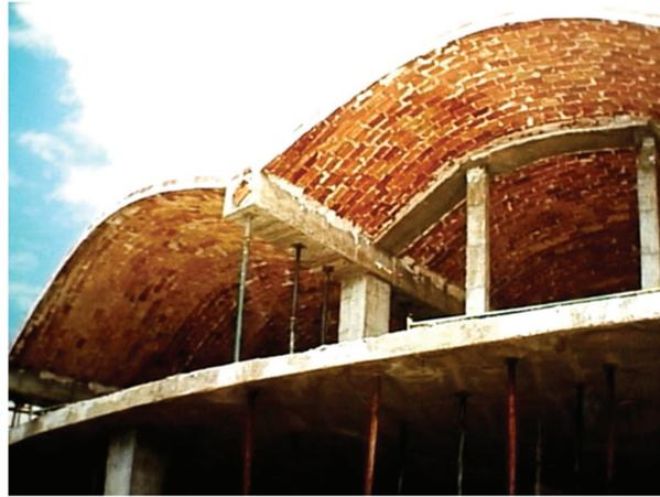
**Figure 27.** Vault pieces are constructed in hollow thin brick with steel mesh for reinforcement and attached to a concrete frame.
