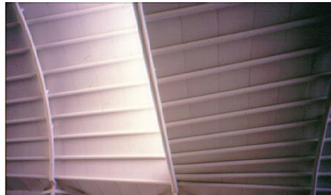
**Figure 23.** Interior view showing light diffusion at the central conoid. School of engineering of Sevilla.
