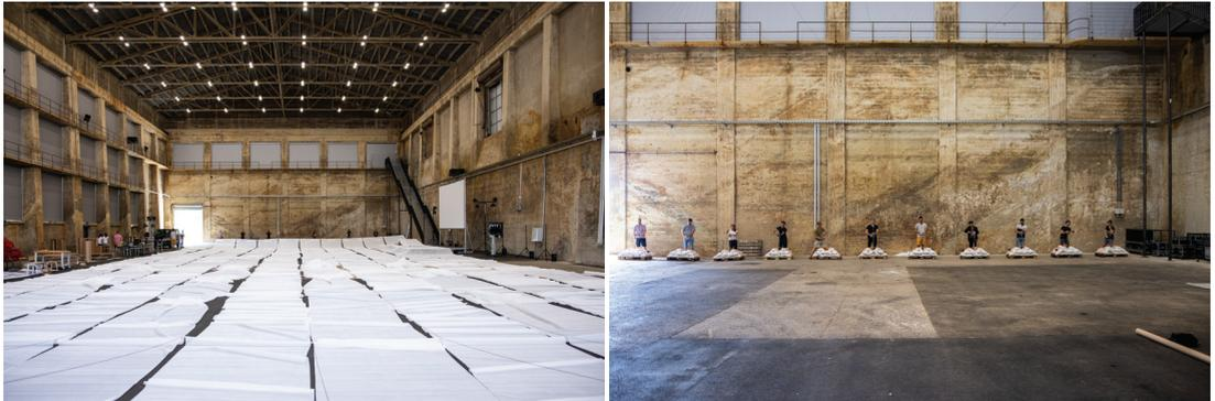
**Figure 15.** The 10 fabric strips were first unrolled on the ground and connected to the cables (a). The entire system was later lifted into the final position through a set of hand-operable winches located at the ground level (b). Photos by Shuaizhong Wang.
