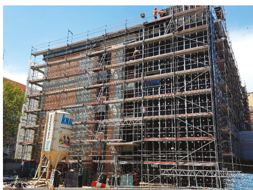
Figure 7. Example of façade scaffold with an area of 300–600 m 2 (authors' archive).
