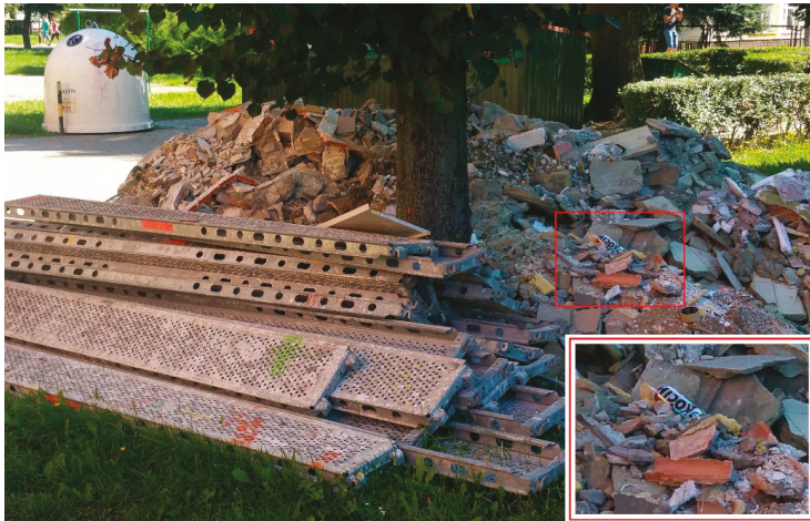
Figure 14. Beer can in the assembly yard at the examined construction site (authors' archive).
