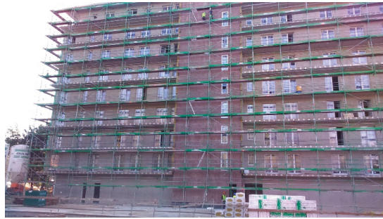
Figure 9. Example of façade scaffold with an area of 900–1500 m 2 (authors’ archive).
