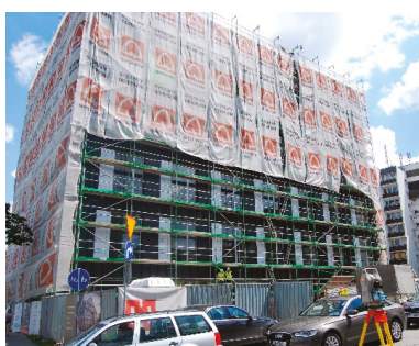
Figure 8. Example of façade scaffold with an area of 600–900 m 2 (authors' archive).
