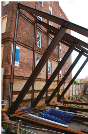
Figure 18. Temporary steel bracing of the strut-cantilever type (photograph by the authors).
