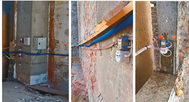
Figure 7. HLC system for baseline measurements with data transfer to the GETEC server (photograph by authors).
