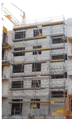
Figure 6. Example of façade scaffold with an area of 30–300 m 2 (authors' archive).
