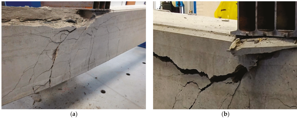
Figure 11. Failure of HPC beam: crack pattern (a), and rupture of the compressed part of the cross-section (b).
