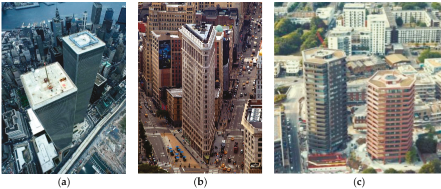
Figure 2. Three example pictures of: (a) rectangular plan building (WTC buildings, New York, USA) [23], (b) triangular plan building (Flatiron Building, New York, USA) [24] and (c) hexagonal plan (Hoxton Press towers, London, UK) [25].
