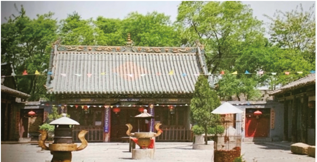
Figure 10. Main Hall/Sacrificial Hall.
