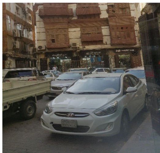
Figure 27. Narrow alleys turned into car parking.
