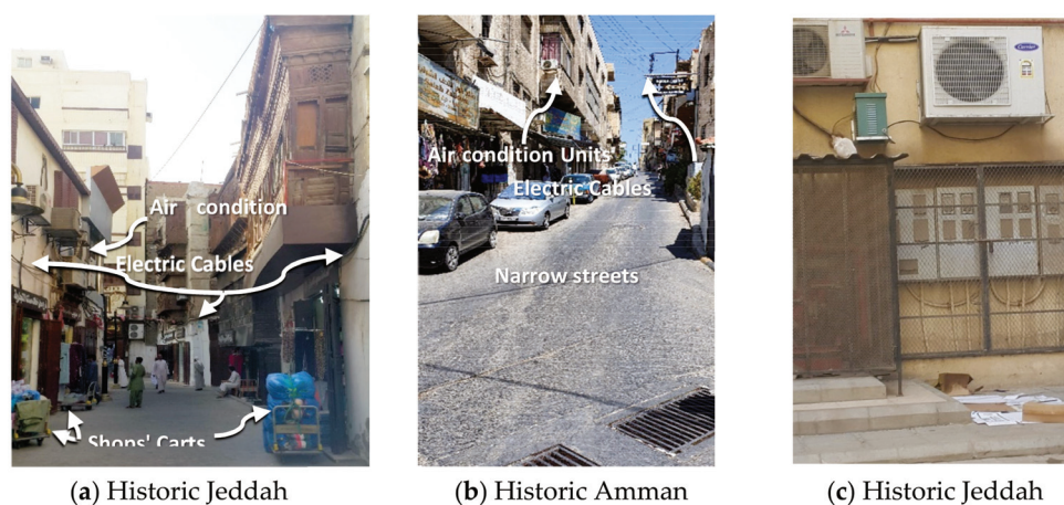
Figure 2. (a) Services in historic Jeddah alleys, (b) services in the historic area of Amman, (c) outdoor electric systems in historic Jeddah.
