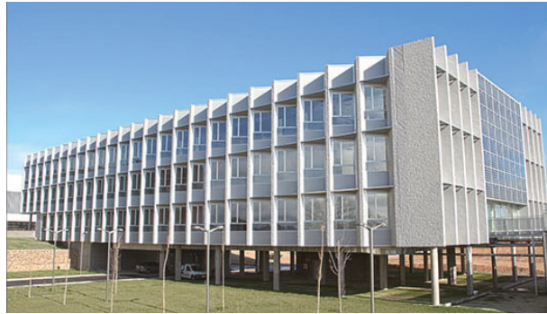
Figure 1. General view of the LUCIA building.
