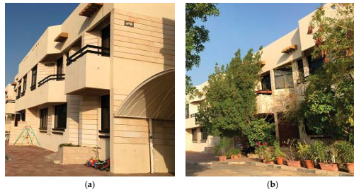
Figure 1. Plant-shaded façade in comparison with unshaded façade of identical housing units, Al-Ain, where (a) Unshaded building façade (bare wall), (b) Plant-shaded façade (plant-shaded wall).
