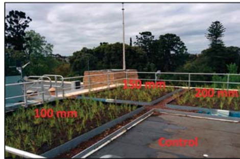
Figure 17. The experimental green roofs at The University of Melbourne's Burnley Campus in December 2015 with sparse (20% cover) vegetation.
