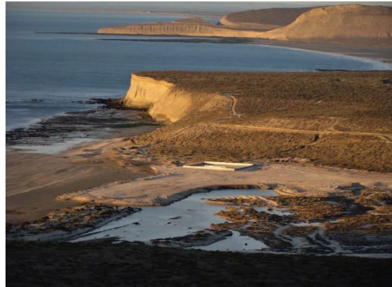
Figure 4. Partial rebuilding work of coastal dunes and elevation of coastal terrain.
