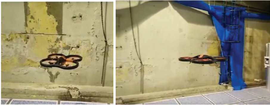
Figure 16. The aerial robot (AR Drone 2.0) during wall inspection.
