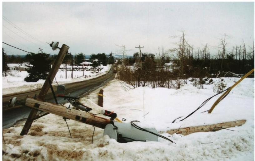
**Figure 2.** Example of icing impact on a medium voltage distribution line (1998 Eastern Canada ice storm, credit: private archive).
