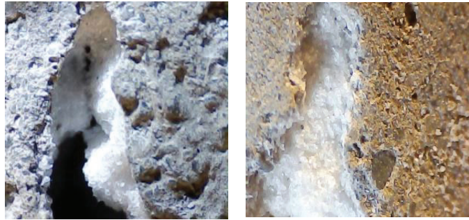
Figure 11. Sealed images of mortar cracks with 6% NC.
