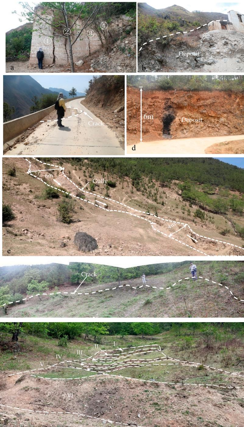
**Figure 6.** Field investigation of old landslide deposits. (a) Cracks on the surface of the house; (b) the downstream boundary of the deposit; (c) a small landslide in the free direction of the highway; (d) a typical section at the top of the downstream side of the KZG Village; (e) the gully between platform IV and platform V; (f) a tension crack in MP landslide; (g) a small soil landslide in MP landslide.
