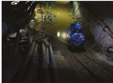
Figure 1. Disaster caused by floor water inrush in a mine working face.
