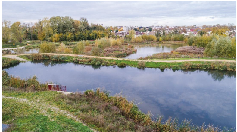
Figure 7. Newly created wetlands: river expands to a larger floodplain, thus preventing flooding in neighbouring settlement while providing habitats for many species © SIAH: Syndicat Intercommunal d’Aménagement Hydraulique of Croult and Petit Rosne.
