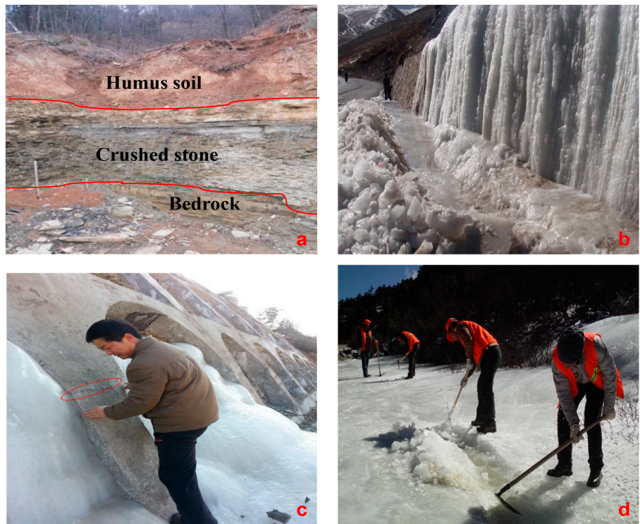
Figure 1. The soil composition and waterfall ice hazards of the research site (a) Soil composition (b) Large-scale highway waterfall ice (c) Facing wall dehiscence induced by waterfall ice (d) Highway waterfall ice extended to the road surface.
