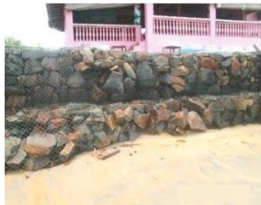
Construction of a protective stone bund in Mboamanga
