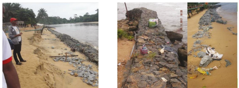
Figure 19. Construction of a protective dyke at the Lobé waterfalls in Kribi. (Credit: Mbevo, 2017; Tchindjang, 2013).
