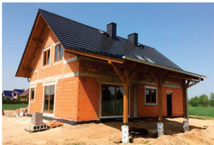
Figure 5. The analyzed building constructed with traditional materials.
