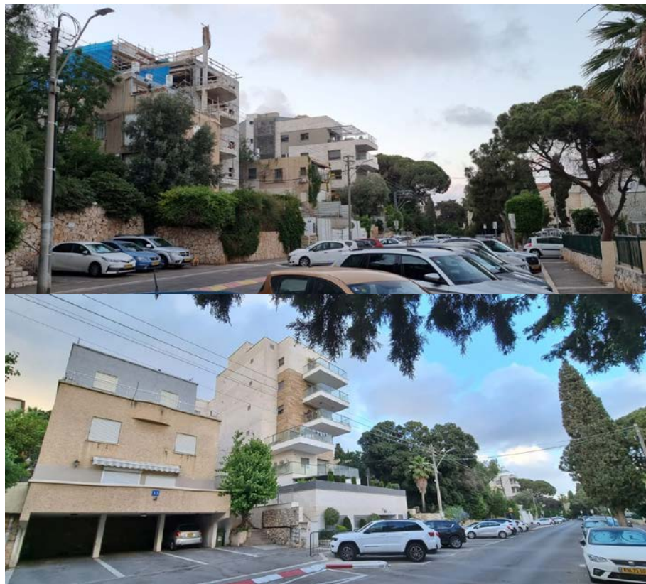
Figure 7. De-Israeli site, during the transformation of TAMA38 construction. A view from the inner side of the site. Photographed by the author, 2022.
