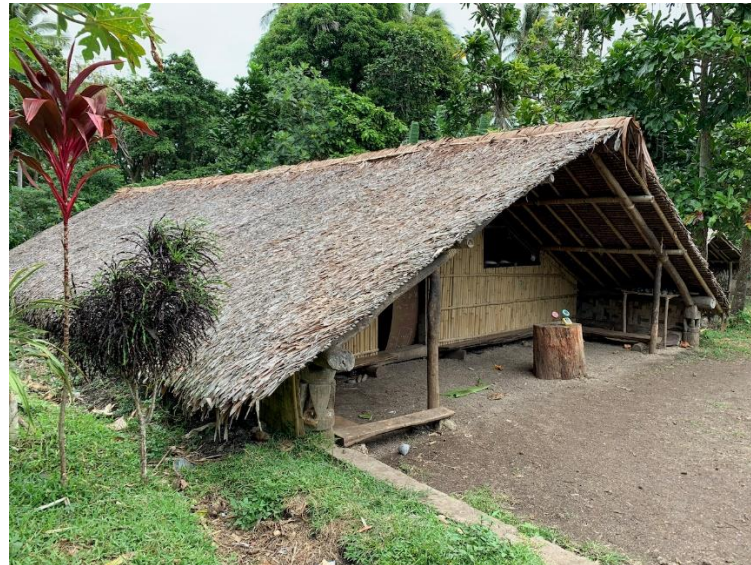
Figure 3. An improved version of a traditional house in Maewo that was built after training by CARE (photo credit: Jen Bowtell).
