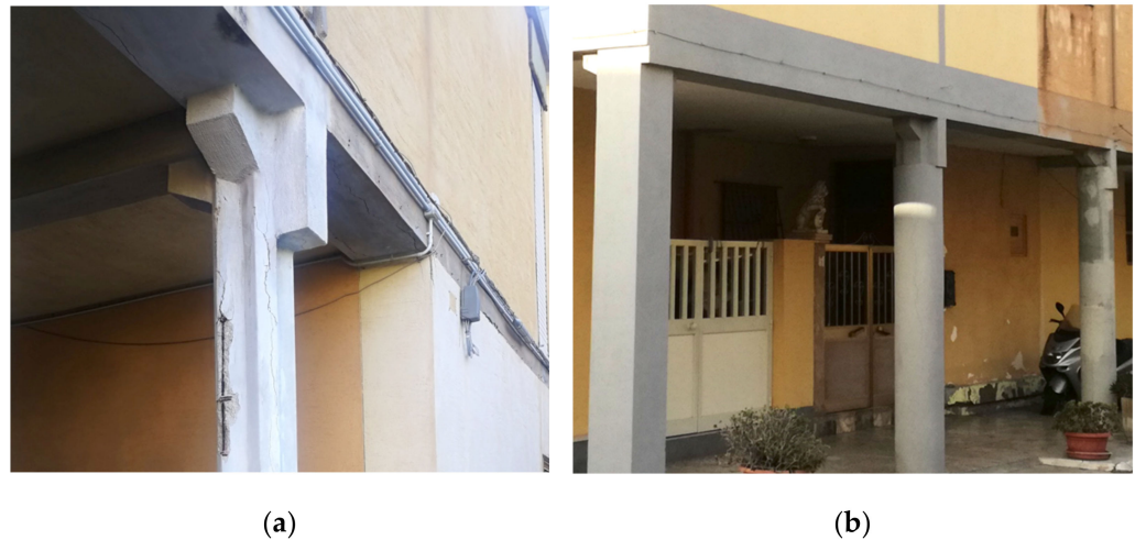
Figure 8. (a) Original shape of pillars designed by Valori. (b) Consolidation of pillars in the portico of court “B”, executed in 2012. Author: Rossella Corrao.
