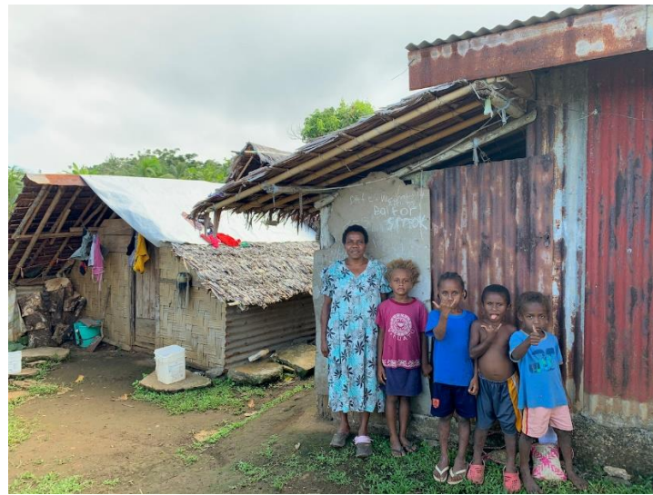
Figure 1. A temporary house built with salvaged materials after TC Harold in Pentecost. The structure on the left has tarpaulin sheets provided as emergency relief by CARE (photo credit: Jen Bowtell).
