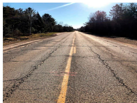
(b) View of the original roadway condition
