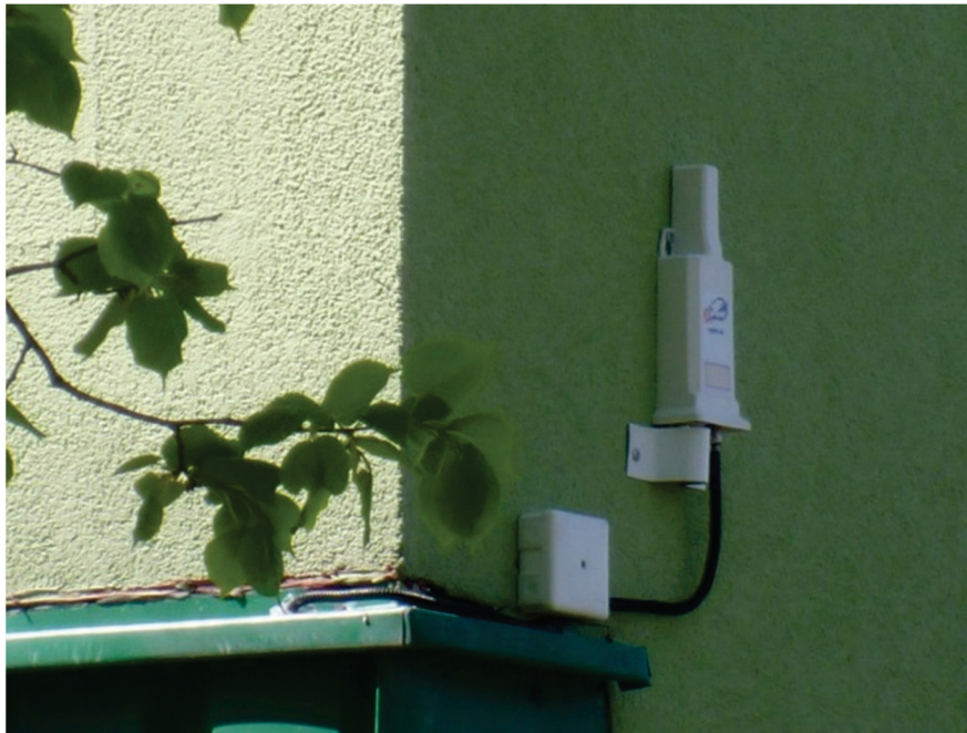
Figure 1. Weather forecast receiver Egain Hub, building A at 12 Śniadeckiego St. in Łomża.
