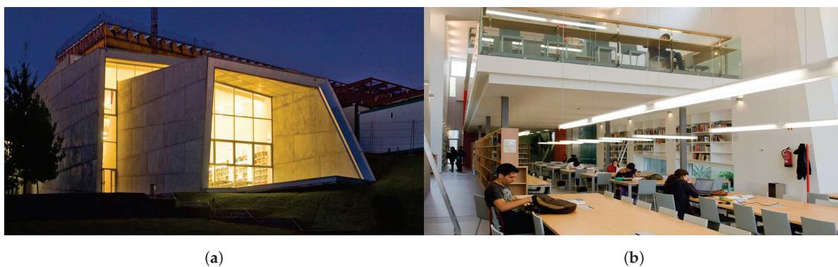
Figure 1. Appearance of the analysed building: (a) exterior and (b) interior.
