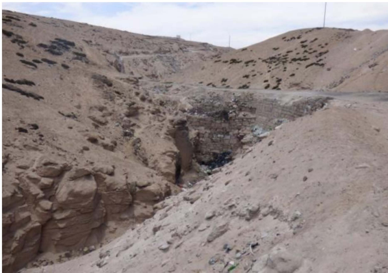
Riverbed of the Devil’s Creek obstructed by an informal em- The place of the informal embankment collapsed by the bankment as an access trail to farms on the Alto de la Alianza flood of 22 February 2020 and that caused the flood to- hill. Source INGEMMET (2016). wards the city of Tacna.
