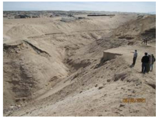
Riverbed of the Devil’s Creek obstructed by an informal em- The place of the informal embankment collapsed by the bankment as an access trail to farms on the Alto de la Alianza flood of 22 February 2020 and that caused the flood to- hill. Source INGEMMET (2016). wards the city of Tacna.
