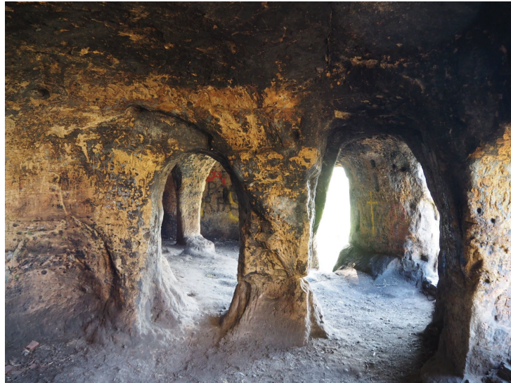
Figure 3. The interior of Anchor Church (Derbyshire): Although thin internal rock walls have been partly removed, features such as tall narrow Romanesque doors and a debased pilaster relate to the initial construction of the structure. Photograph E.R Simons.
