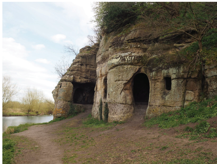
Figure 2. Anchor Church, Derbyshire, is a probable early medieval hermitage adapted and used in the eighteenth and nineteenth centuries, but with little change to the fabric. Photograph E.R Simons.
