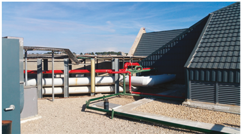
Figure 11. Roofing and installations (Maintenance Indicator = 2.5).
