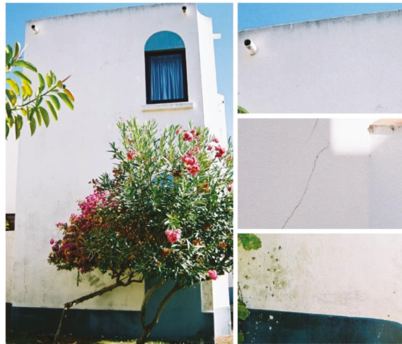
Figure 1. First case study: rendered façade (data sourced from Reference [46]).
