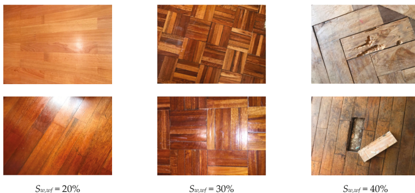
Figure 3. Illustrative examples of the overall condition of the wood floorings for different levels of the severity of degradation index.
