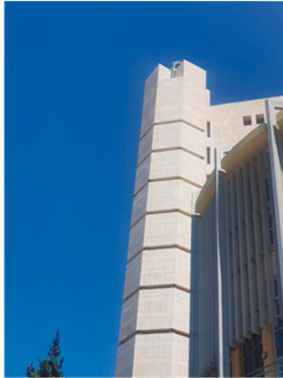
Figure 10. Exterior envelope (Maintenance Indicator = 2.5).
