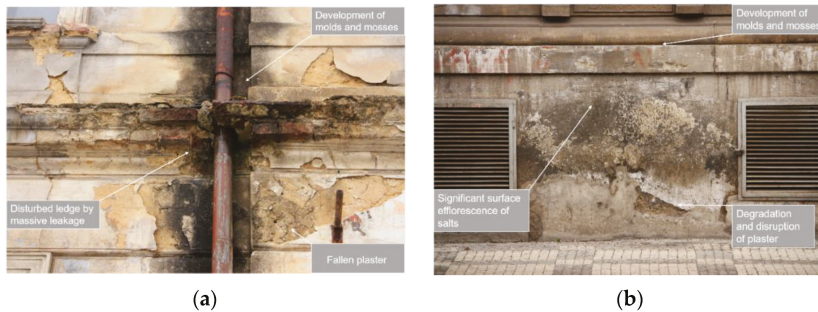
Figure 2. Images clearly showing the most common failures of structures from the second half of the 19th and the early 20th centuries caused by degradation processes initiated in these cases by the combination of moisture, an incorrect design solution and neglected maintenance. The following are clearly visible on images: (a) fallen plaster, damaged ledge by massive leakage, mold and mosses; (b) degradation and disruption of plaster, significant surface efflorescence of salts, mold and mosses.
