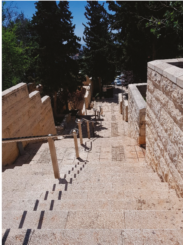
Figure 12. Stairs and drainage infrastructures around the building (Maintenance Indicator = 2.75).
