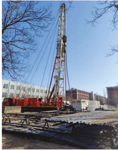
Figure 22. The process of Renre 4 well unblocking operation.
