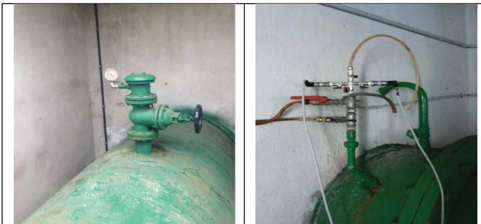
**Figure 2.** Typical TM branches where the inaccessibility is evident: the only appurtenance is just upstream of an inaccessible tunnel.
