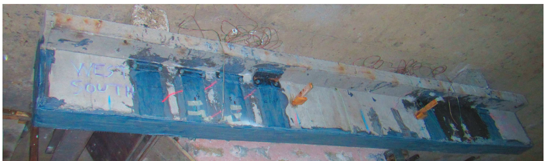
Figure 21. The 3rd strengthening scheme. Open hoop CFRP strips with mechanical anchors at the West part and closed hoop anchor ropes at the East part (The same as in Strengthening scheme 2). The flexural upgrade of the 3rd strengthening scheme consisted of five (5) CFRP layers (each 0.131 mm thick and 120 mm wide) attached at the bottom side of the T-beam specimen.
