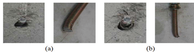
Figure 9. Failure mode for static shear tests: (a) M10 set anchor; (b) M12 set anchor.
