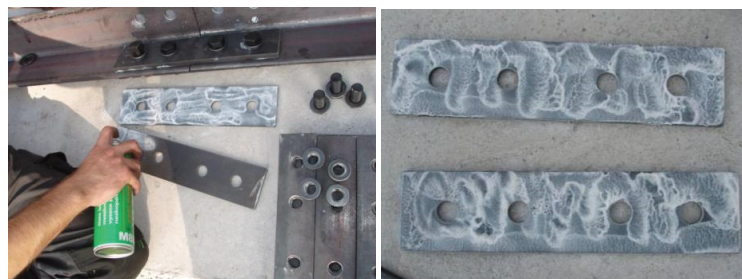
Figure 9. Application of Teflon Vaseline to the splices.
