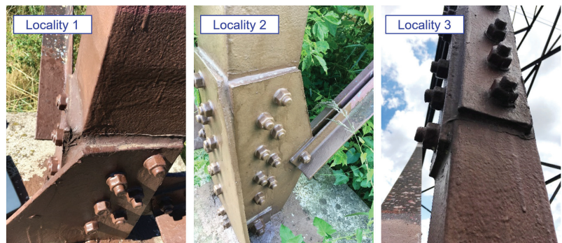
Figure 18. Functional crevice protection with sealant (selected examples).
