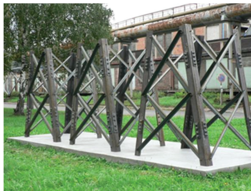
Figure 7. View of the experimental towers' assembly at the time of installation.
