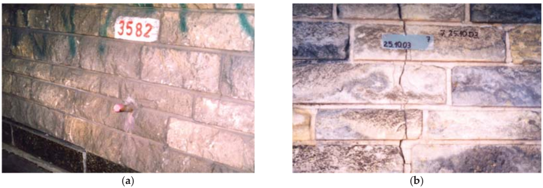
Figure 2. Applied monitoring of the impact of the investment projects on neighboring facilities: (a) measurement benchmark; (b) sealant for observation of crack development.
