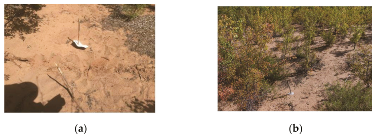
Figure 22. Crack manual management process: (a) Filled cracks; (b) Ecological restoration.
