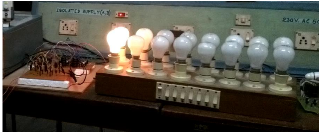
Figure 17. Resistive (Lamp) Load Connected to the Transformerless Inverter.
